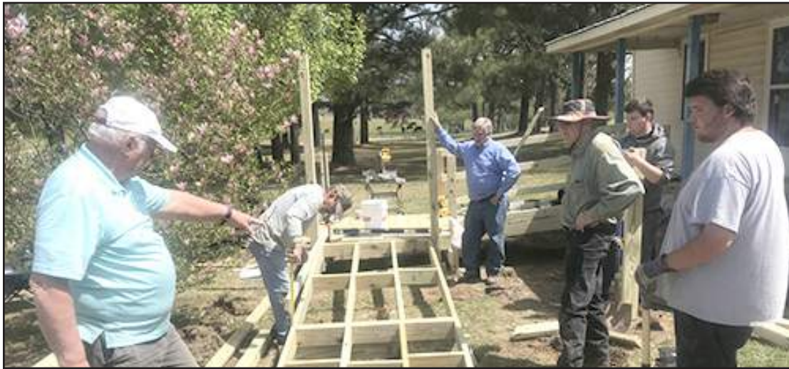
34-A Wheelchair Ramp Service Project
